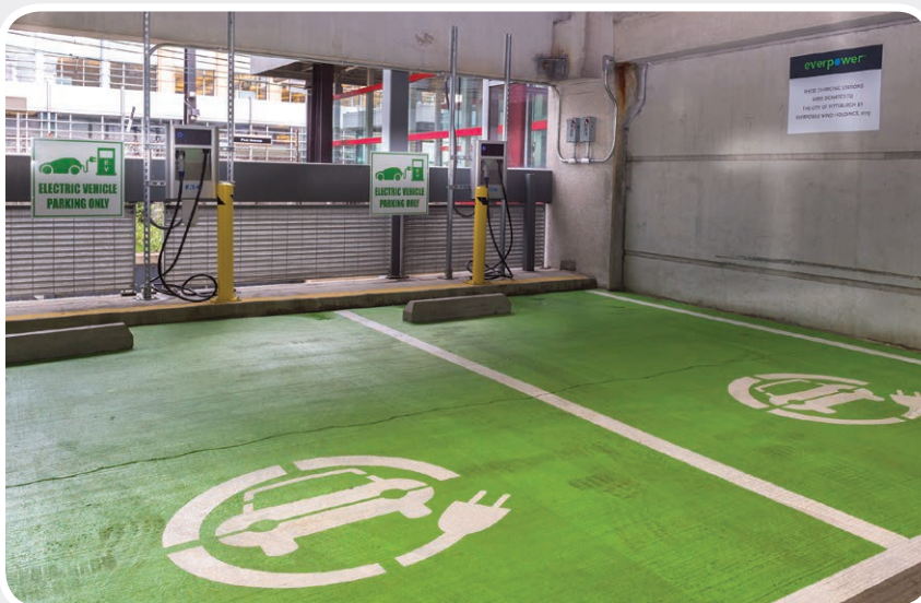
Two Authority garages now house charging stations for the free use of customers driving electrically powered vehicles. A four-hour connection delivers a full battery charge.
